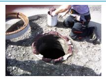
+5°C (+41°F). Pour the complete contents of the component B into the component A container and mix the combined components together thoroughly with an electric stirrer (e.g. drill with mixing blade Collomix WK 70) with at least 500 rpm. The stirring time for the small containers is at least 3 minutes, for the large containers,
