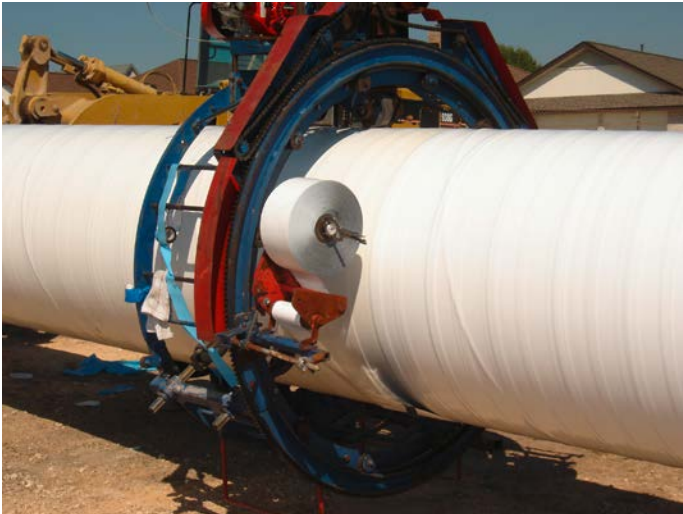
Seal For Life Industries: Pipeline CAT coating.
