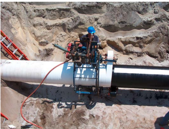
Seal For Life Industries: Pipeline CAT rehabilitation.
